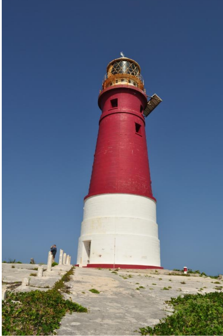
Figure 3.24 Photo of Hole in the Wall Lighthouse
